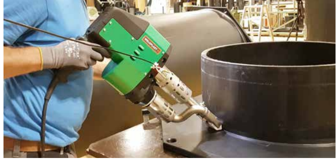
The powerful WELDPLAST S4 in use
