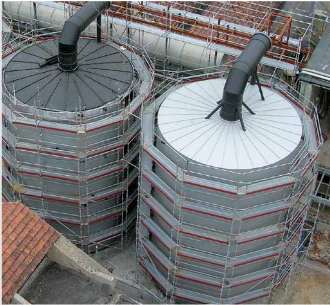
Air purification system, Spain. Material: HD-PE
