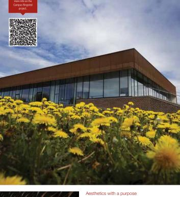
Form and functionality meet when expanded metal is part of the equation, as can be seen from the facade and sun screens for this sports hall. The expanded metal offers creative freedom, as you can choose from various materials and different types of surface treatments to make the metal suit the overall architectural purpose.
