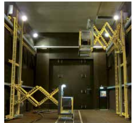
Scissor-type lifting platform in a blast booth
