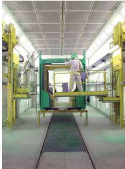
Swivelling lifting platform in a combined paint-spraying and drying booth
