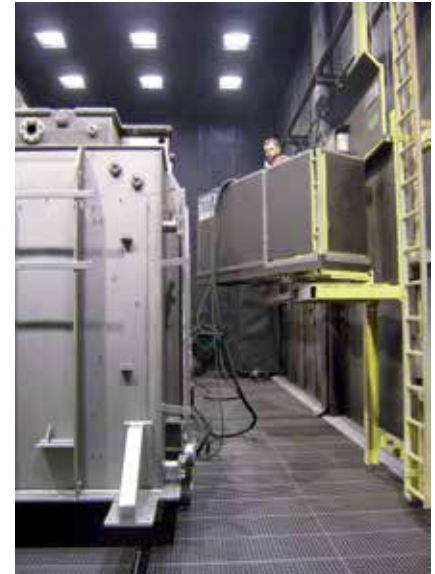
Swivelling lifting platform in a blast booth
