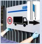
In vertical adhesive bondings, e.g. attaching panelling elements to walls, the bonding is exposed to shear stress. Due to this, the major part of the load should be close to the adhesive surface, so the load does not generate peel or split tensile strength.
