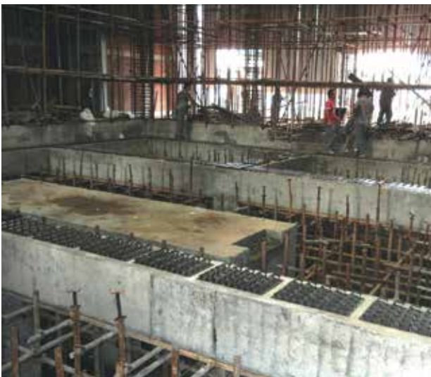
Spring mounts being installed for floating floor system
