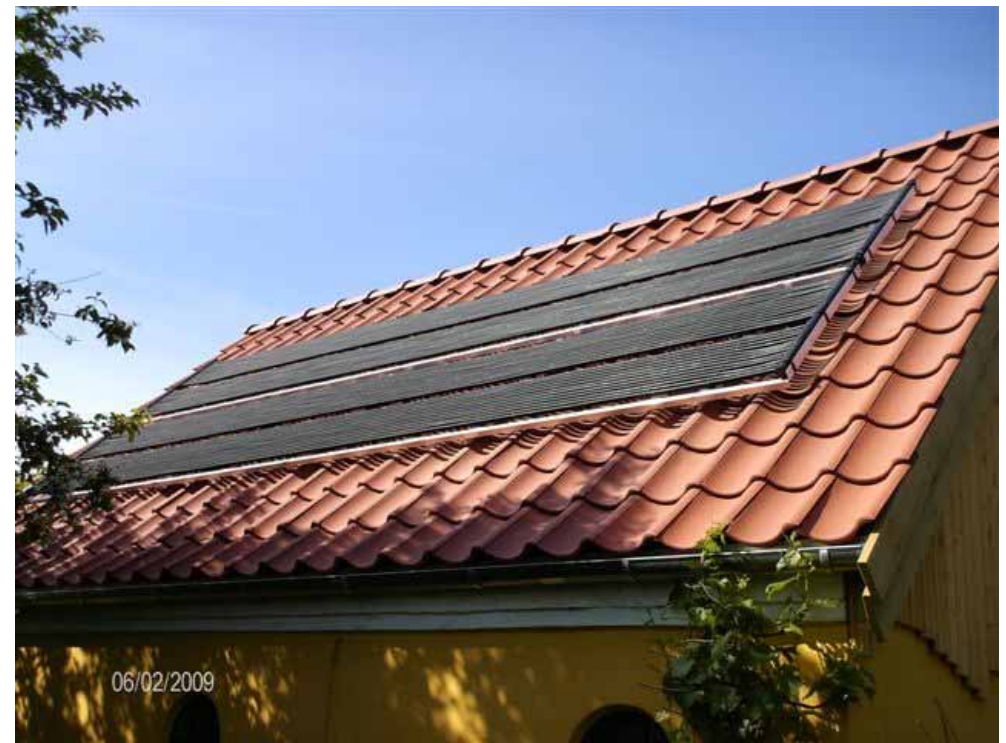
Assembling on the ground and then put up on the roof
