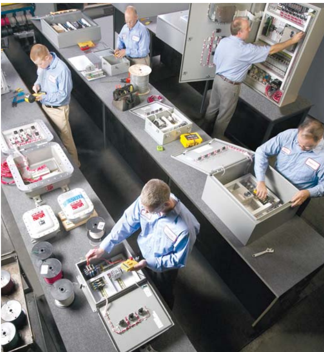
Panel assembly area of Controls Department
