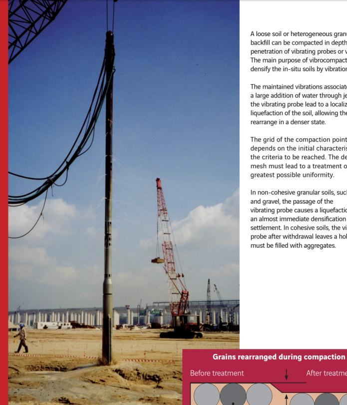
A loose soil or heterogeneous granular backfill can be compacted in depth by the penetration of vibrating probes or vibroflots. The main purpose of vibrocompaction is to densify the in-situ soils by vibration.
