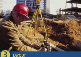
The LM80 graphically guides you through your building layout, navigates you to your critical building alignments, and creates as-built records of all layout points. You can also use the LM80 to inspect the location of building elements once they are installed.
